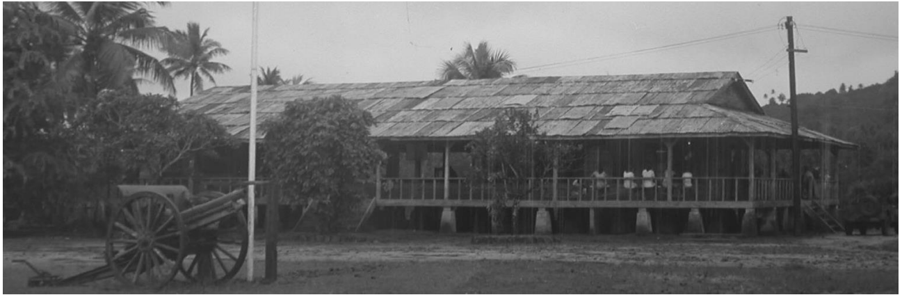
Figure 78. Similar Japanese barrack at the naval headquarter at Iasiring, Nett, which was used as US Naval Administration Building in 1945 (courtesy of Micronesian Seminar, Naval Historical Center Collection, NHC04109). 13
