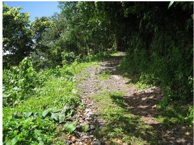
Figure 6. The steep road from the second parking area.
