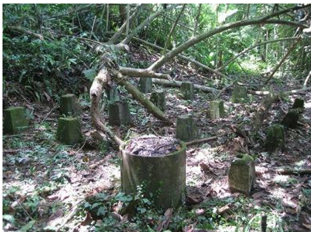
Figure 65. Concrete foundation posts.
