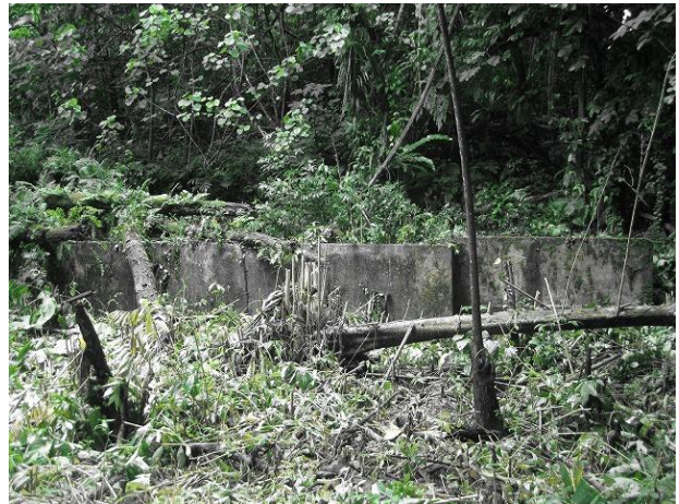
Figure 37. Two concrete water-cooling tanks and fuel storage tank
